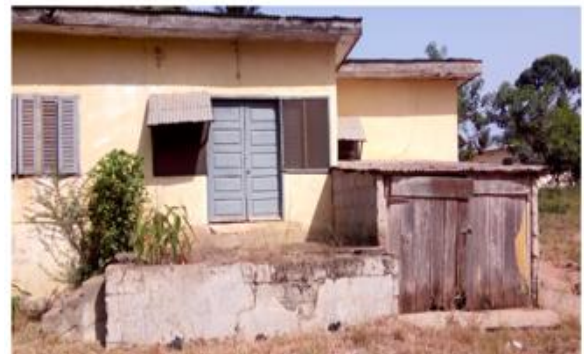
Fig. 8. Staff residence for Ejisuman Senior High School. Source: Author's field survey, 2017.
