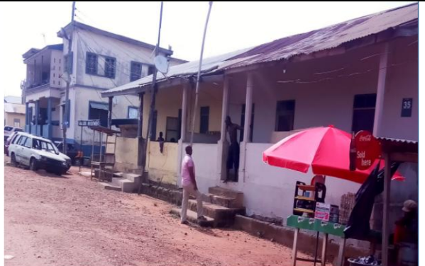
Fig. 11. Staff residence for the Police Service in Ejisu. Source: Author's field survey, 2017
