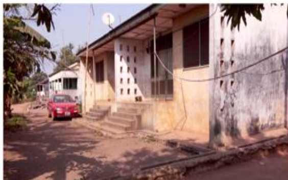
Fig. 3. Staff Residence of Railway Authority in Ejisu. Author's Source: field survey, 2017.
