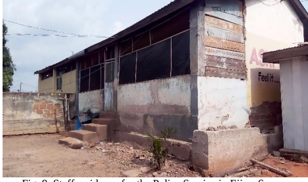
Fig. 9. Staff residence for the Police Service in Ejisu. Source: Author's field survey, 2017
