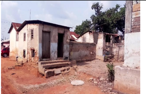
Fig. 10. Staff residence for the Police Service in Ejisu. Source: Author's field survey, 2017
