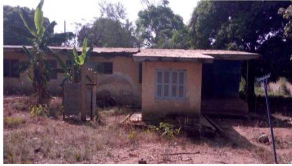
Fig. 6. Staff residence for Ejisuman Senior High School. Source: Author's field survey, 2017.
