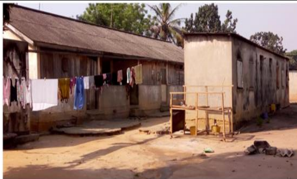
Fig. 2. Staff Residence of Railway Authority in Ejisu. Source: Author's field survey, 2017.
