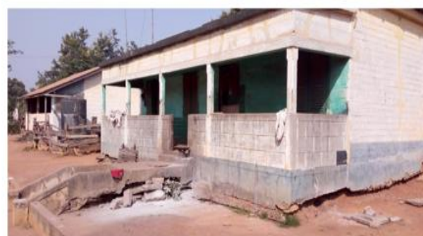
Fig. 4. Staff Residence of Railway Authority in Ejisu. Source: Author's field survey, 2017.
